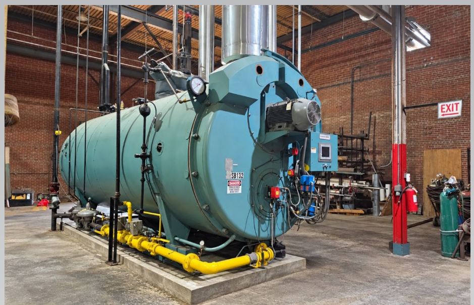
Cleaver Brooks CB Packaged Boiler , Model CBI-700-800-150, Year 1996, S/N CL095976, Max Pressure 150ST PSI, 32,858,500 BTU/Hour, 27,000 lbs./hour
